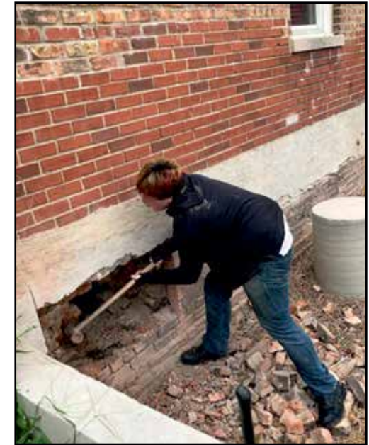
Construction of the Cornerstone Café
